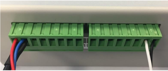
ES Intelli “Ultra” wiring at Controller
